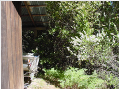
Residence building prior to fuel treatment efforts.
